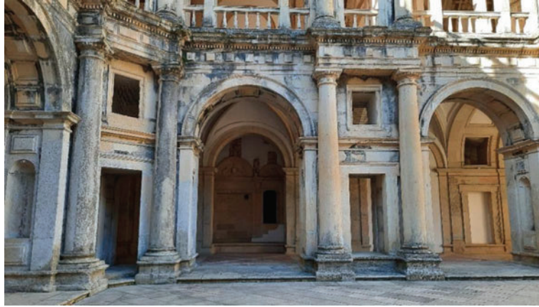
Fig. 10.1 South elevation of the Main Cloister of Convent of Christ in Tomar
